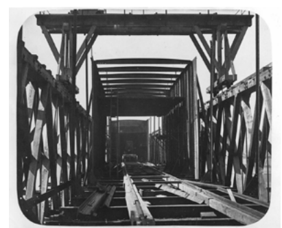
Fig 6. William Notman, Framework of Tube and Staging Looking In, Victoria Bridge , Montreal, 1859. Notman famously photographed the construction of this new bridge linking Canada and the US.
