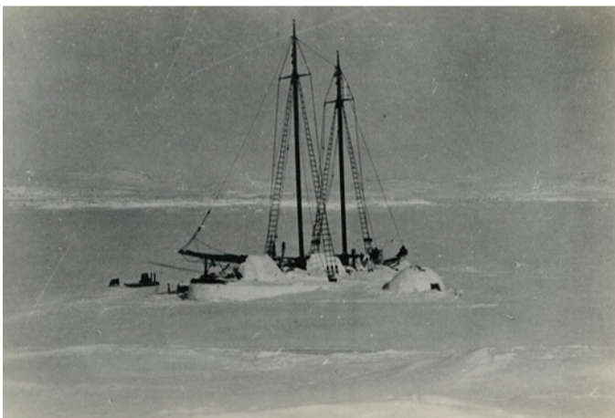
LEFT: The schooner Bowdoin at Idjirituq (Schooner Bay) during the winter of 1921-22. The crew worked with local Inuit to construct snow domes over the boat's hatches; the domes provided wind protection while allowing air to circulate into the vessel. Photograph by Donald Baxter MacMillan. RIGHT: The camp of Pitseolak's uncle Kavavow at Idjirituq in the winter, c. 1921-22. Photograph by Donald Baxter MacMillan.
