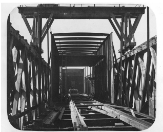
William Notman, Framework of Tube and Staging Looking In, Victoria Bridge, Montreal, 1859 Silver salts on paper mounted on card, albumen process 23 x 28 cm
