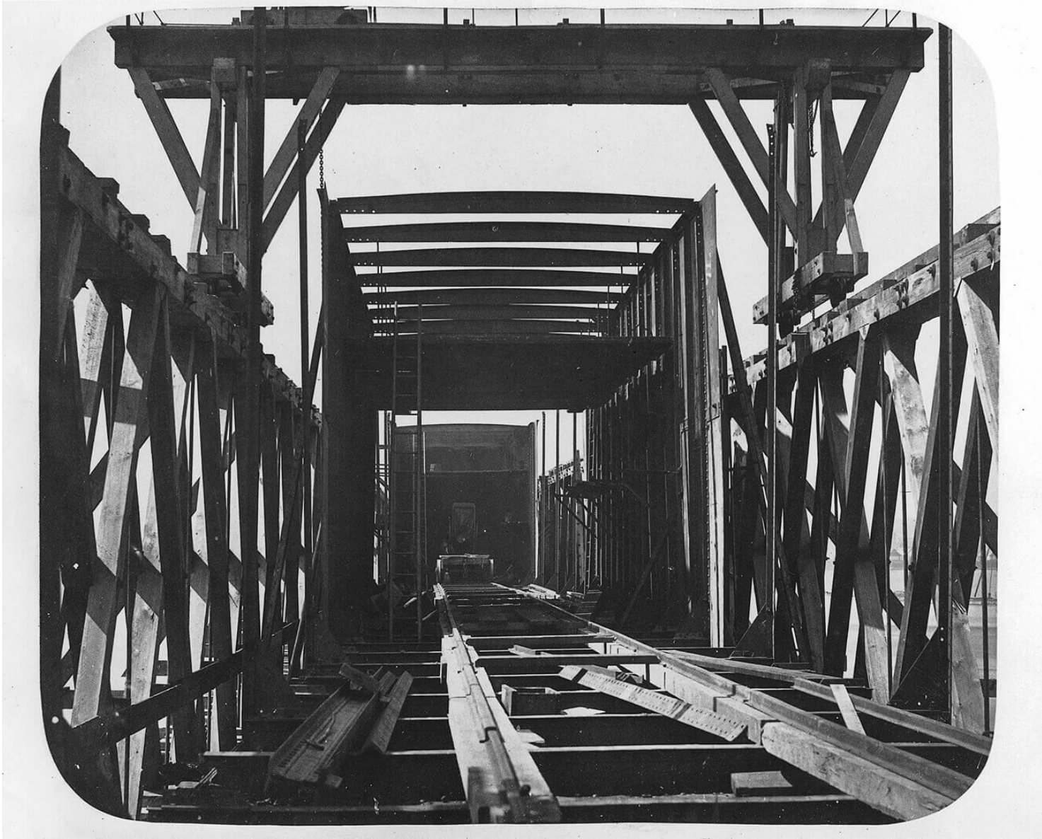
William Notman, Framework of Tube and Staging Looking In, Victoria Bridge, Montreal , 1859
