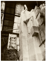
Temporary protective structure at the top of the Vimy Memorial pylons, n.d., photographer unknown. Walter Seymour Allward Fonds, Queen's University Archives, Kingston.
