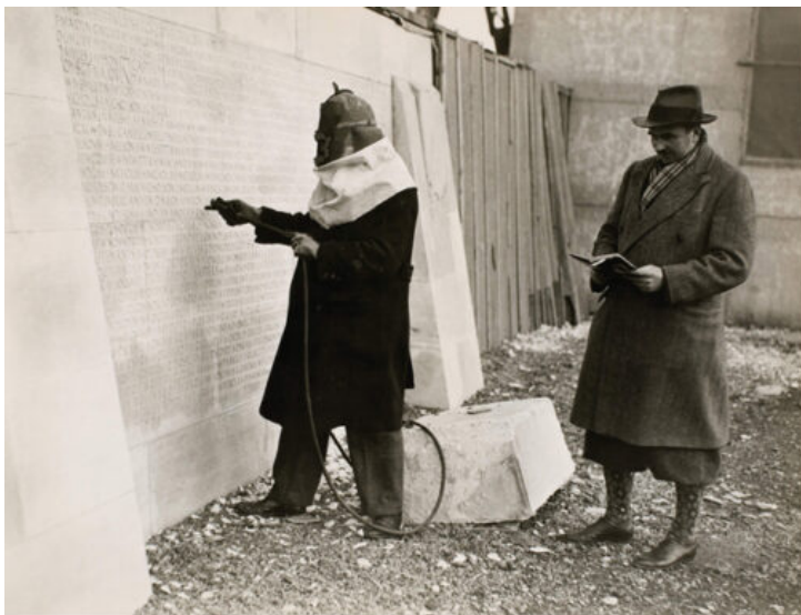
LEFT: Sandblasting names onto the lower wall of the Vimy Memorial, n.d., photographer unknown. RIGHT: Two men cutting names on the Vimy Memorial, n.d., photographer unknown.
