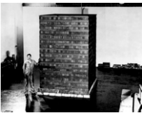
Chicago Pile-1 (Graphite Lattice), 1942, photographer unknown. Collection of the United States Department of Energy (HD.5A.024). Courtesy of the United States Department of Energy, Historian's Office.
