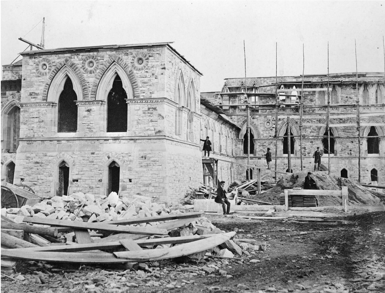
Samuel McLaughlin, Parliament Buildings under construction, centre block, rear view , c.1862, 28.7 x 37.7 cm, Library and Archives Canada, Ottawa.
