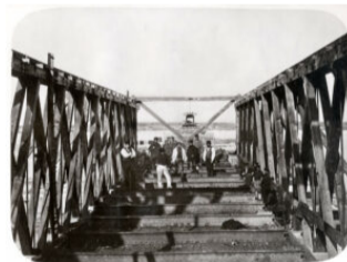
William Notman, Framework of tube and staging no. 8, Victoria Bridge, Montreal, QC, 1859 Silver salts on paper mounted on paper 22 x 29 cm
