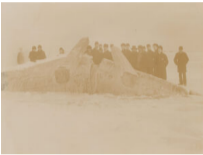
Waterworks upheaval , 1893, by F.W. Micklethwaite. Collection of the City of Toronto Archives (Fonds 200, Series 376, File 1, Item 29a). Courtesy of the City of Toronto Archives.
