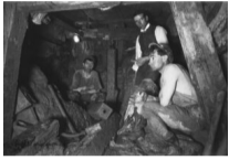
Storm overflow Sewer, Barton Avenue , June 5, 1912, by Arthur Goss. Collection of the City of Toronto Archives (Fonds 200, Series 372, Subseries 59, Item 47). Courtesy of the City of Toronto Archives.
