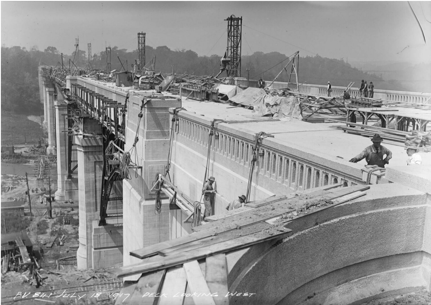
Bloor Street Viaduct, Deck Looking West, July 18, 1917
