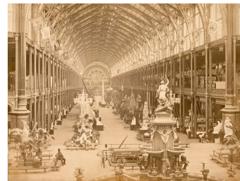
William England, Interior view of the International Exhibition, London, 1862 , photograph, dimensions undefined, Science Museum Group, London.
