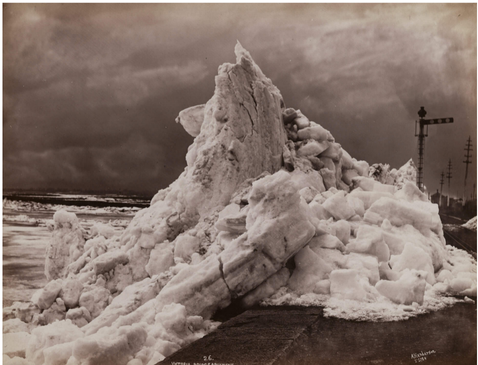
Alexander Henderson, Victoria Bridge. Abutment, Ice shove , c.1887, albumen print, 15.3 x 20.2 cm, Library and Archives Canada, Ottawa.
