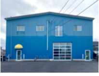
Exterior of 2482 Maynard Street, home to The Blue Building Gallery, Halifax, 2021. Photograph by Ryan Josey. © Ryan Josey.
