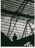
Untitled [Construction, Glasgow], 1928-38. Collection of The Hidden Lane Gallery, Glasgow. Courtesy of CentroCentro, Madrid. © Joseph Mulholland, Glasgow.
